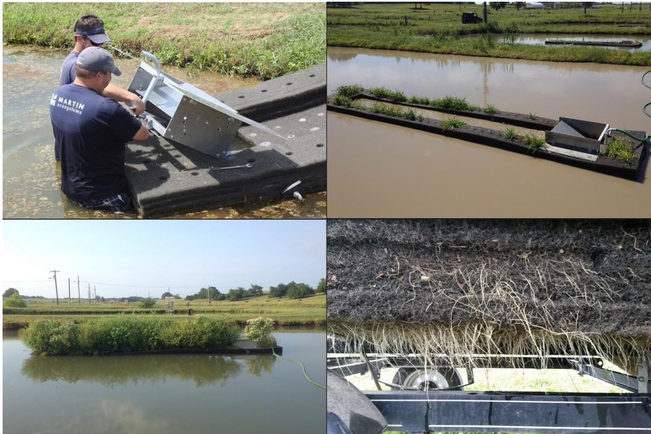
**Figure 1.** Installation of directional airlift system to streambed of FSW (top left), view of the on-island streambed (top right), plant establishment (bottom left), and root canopy beneath FSW at study's end (bottom right).
